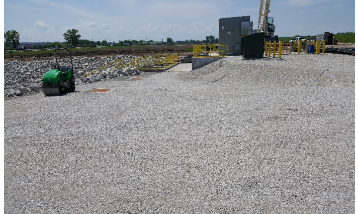
Watershed 4 Pump Station Construction.
