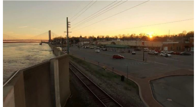
Cape Girardeau Floodwall
