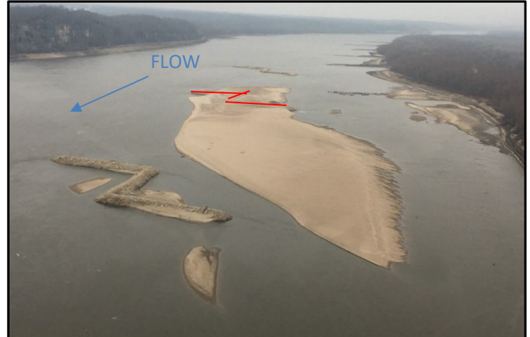
"Z" Dikes constructed under Grand Tower Phase 5 (completed 2017)
