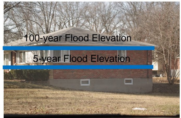
One of 275 at risk homes in the authorized project area. Two drowning deaths occurred across the street from this home in 2008.
