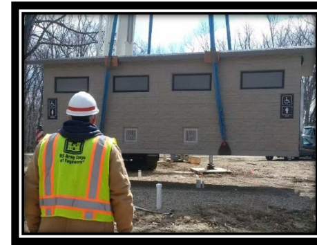
CXT Building being placed
