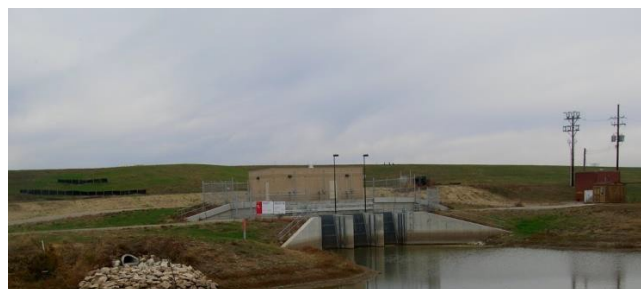
New Chain of Rocks Pump Station
