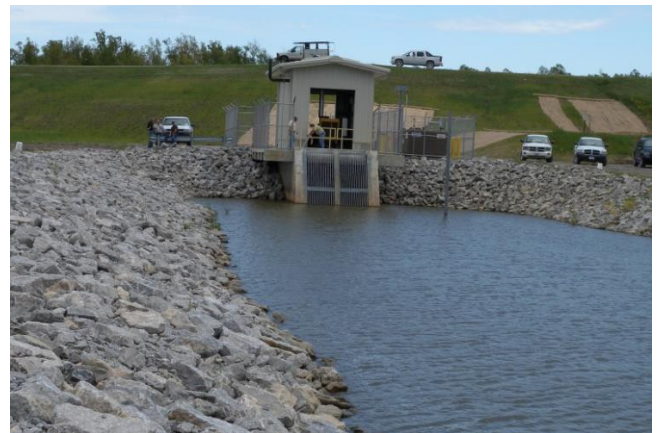
Missouri Chute Pump Station
