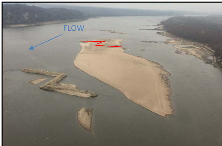
"Z" Dikes constructed under Grand Tower Phase 5 (completed 2017)
