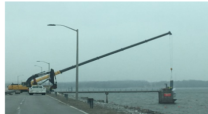
Sluice gate hoist replacement.
