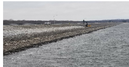
Placement of revetment on upstream shelf.
