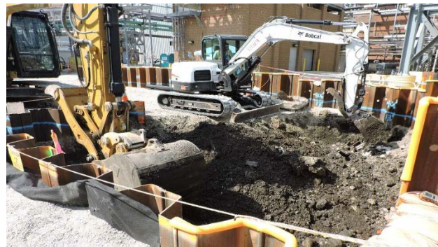
Excavation of contaminated soil at the Mallinckrodt Plant 1, former Building 17 area at St. Louis Downtown Site.
