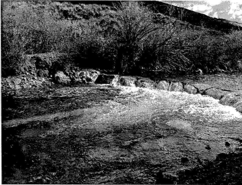
Figure 8. Low-head stone weir on the North Fork of the White River, Colorado
