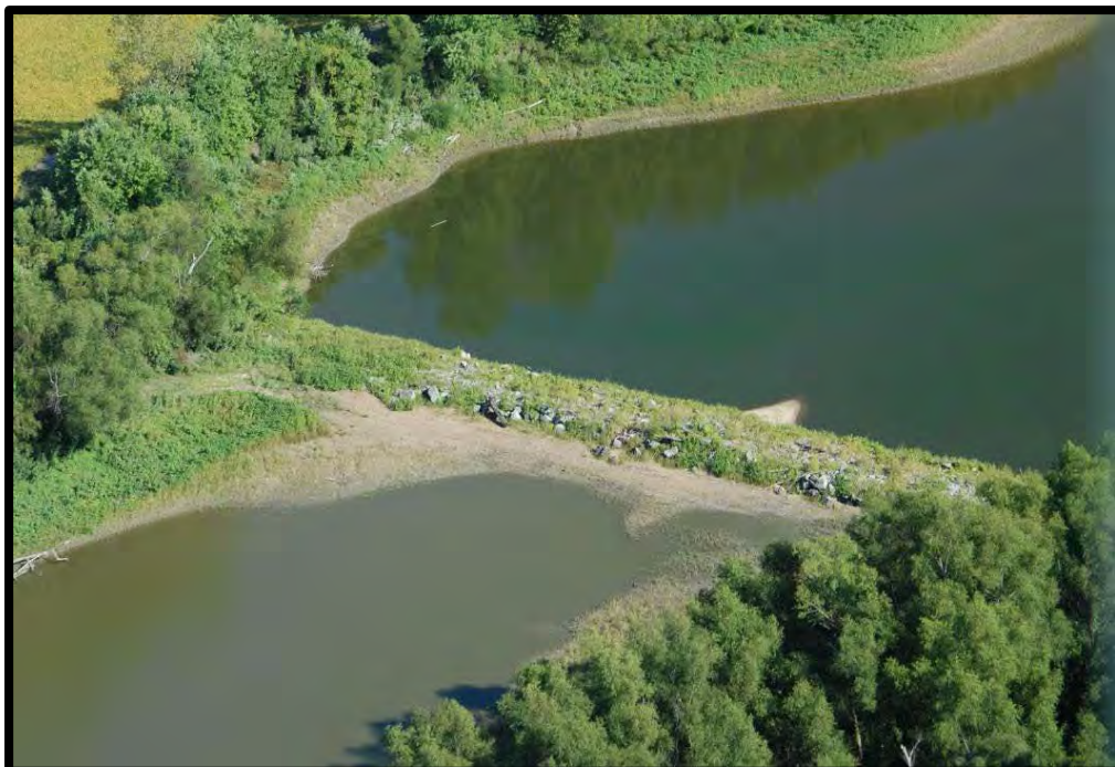
Figure 7. Photo of rock dike/closing structure (7.9L) near the exit of Boston Chute.
