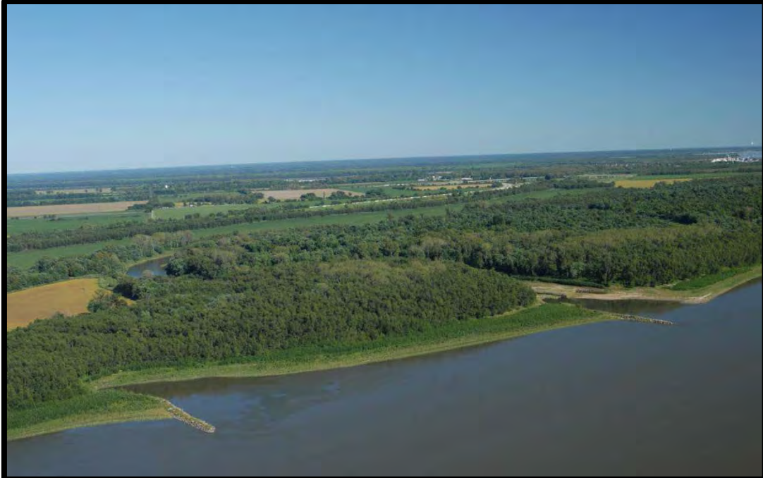
Figure 8. Photo of rock dikes (10.3L) and (10.1L) upstream of Boston Chute.
