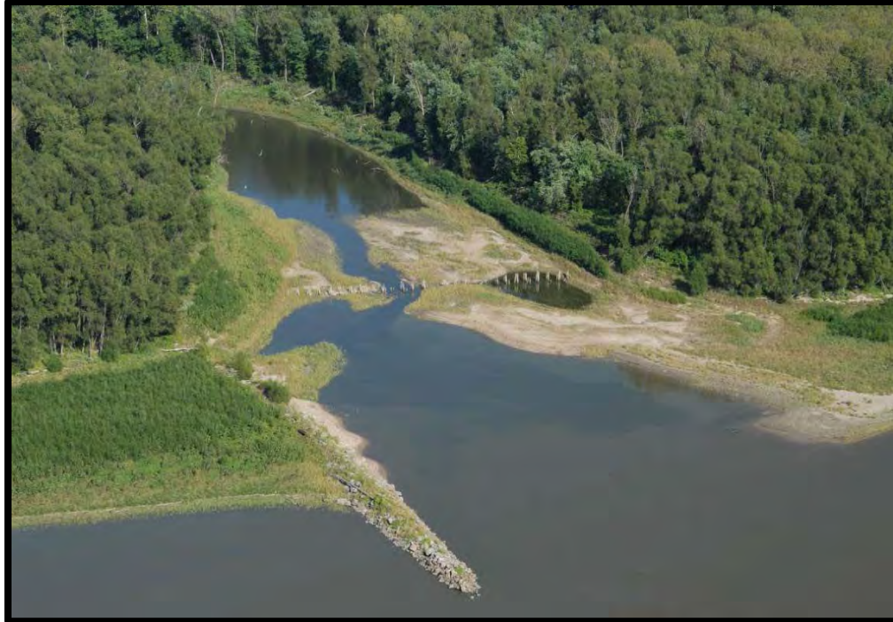
Figure 6. Photo of rock dike (10.1L) and pile dike (10.3L) at the entrance of Boston Chute.
