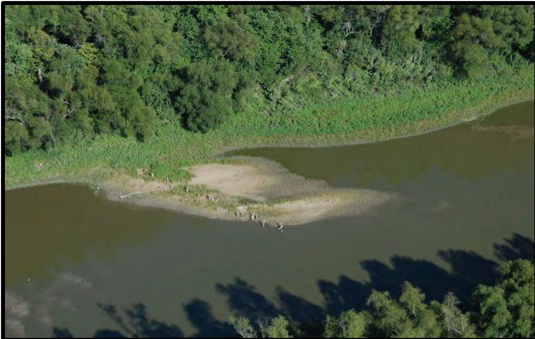
Figure 9. Photo of pile dike (8.2L) near the exit of Boston Chute.
