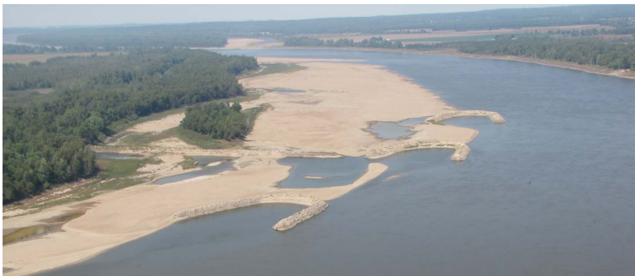
Figure 6. Chevron river training structures near River Mile 32.
