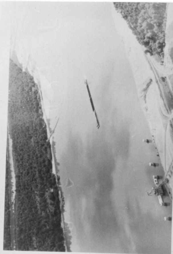
3-2 Aerial view - approx. mile 146.0 showing that new stone dike construction is more effective in trapping materials than pile dike construction. Pile dike is shown in upper left portion of photo.
