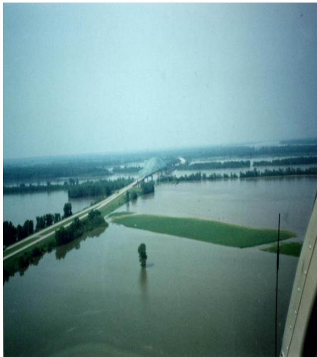
Figure 21: I-57 Bridge During 1993 Flood
