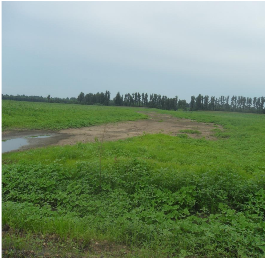
Figure 35: Scour in Low Lying Area of Peninsula after 2011 Flood
