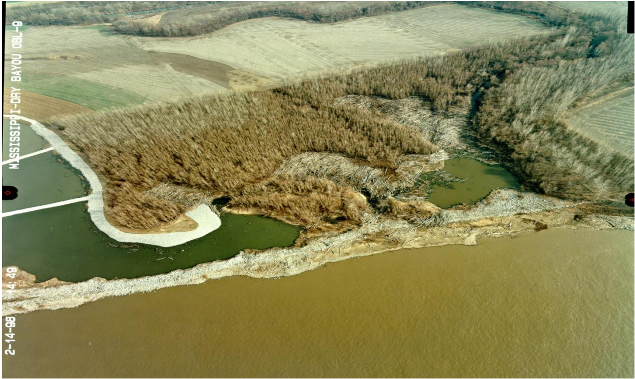
Figure 25: Dry Bayou Revetment February 1998 (demonstrating effective tree screen reducing scour)
