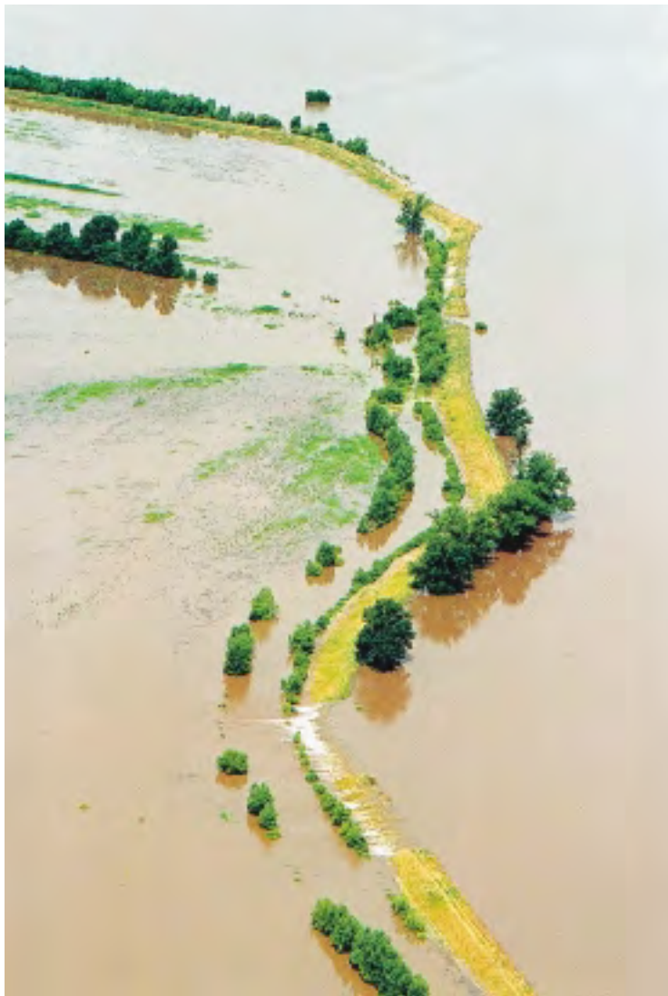
Figure 15-11. Levees were damaged in two ways: from being overtopped as shown here, or from seepage. In either case the levees usually were eroded by the force of the water through the restricted space. Large, deep holes were scoured in the Unimpounded Reach and the Missouri River (Source: St. Louis Post-Dispatch ).
