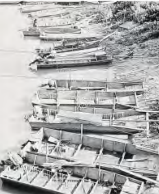
Figure 11-5. These boats display the brail bars used by commercial shellers to collect mussels in the days when the animals were plentiful. The bars, lined with chains and hooks, were dragged along the river bottom where mussels clamped unto the hooks (Source: Richard Sparks, Illinois Natural History Survey, Havana, Illinois).
