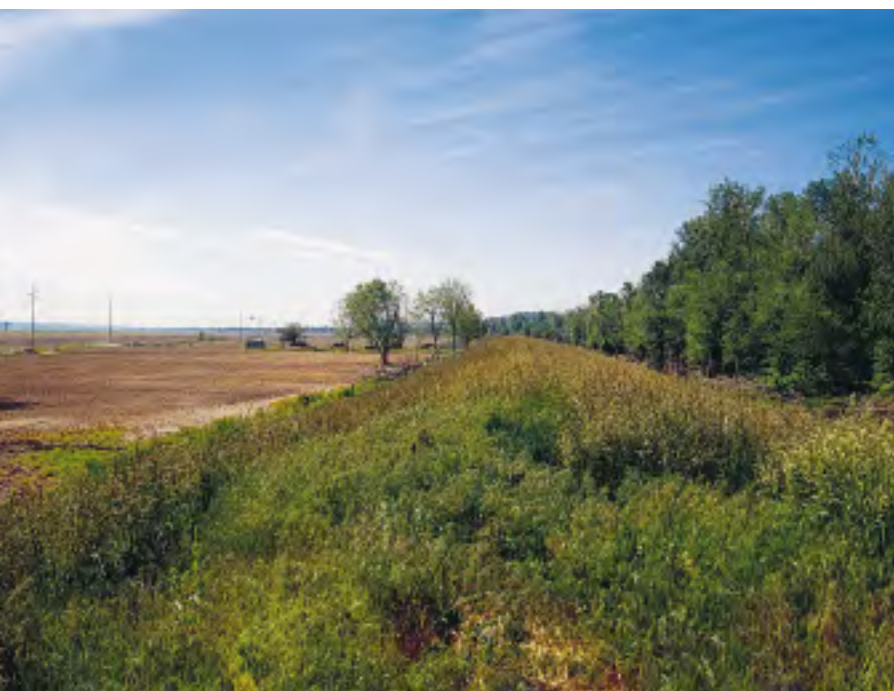
Figure 3-5. The Nutwood Levee is the last in a series that isolates much of the Lower Illinois River from its floodplain.
