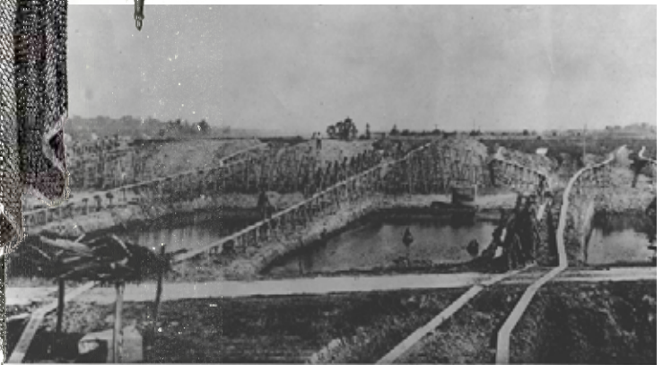
BUILDING LEVEE BY WHEELBARROW
