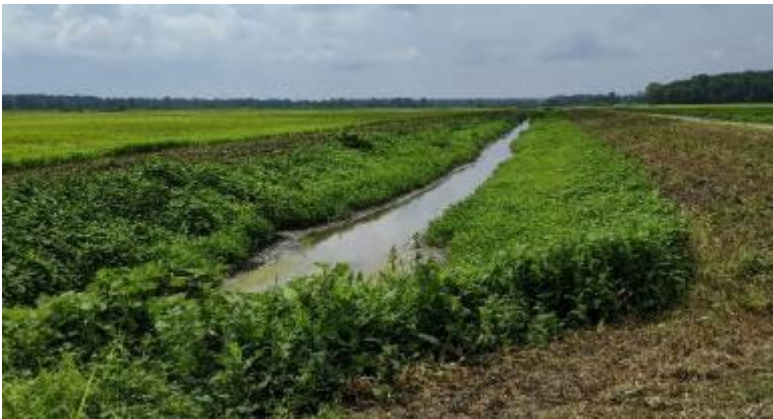
Seepage through berms; sedimentation
