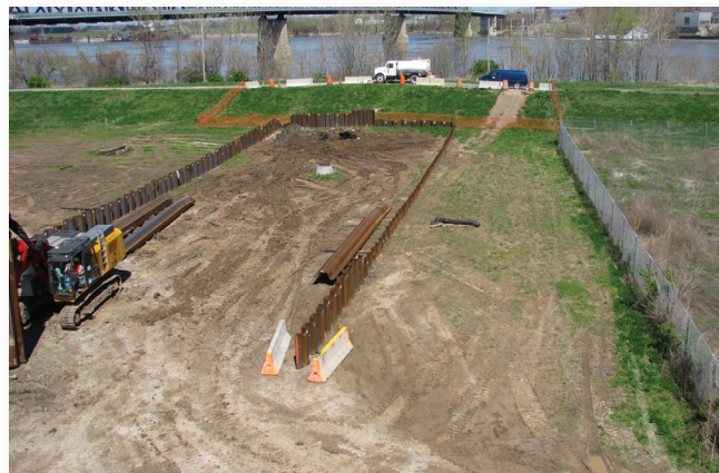
Sheet pile protection system for the City Property excavation is shown nearing completion.
