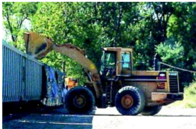
Removal of the final stockpile at HISS is nearly complete. Of the estimated 25,000 cubic yards comprising the Main Pile, roughly 20,200 cubic yards have been removed.
