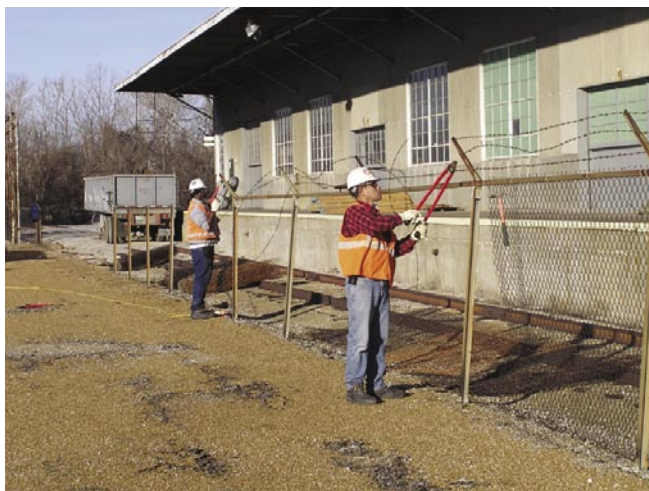
Laborers cut and remove fencing to allow equipment access to contaminated soil.
