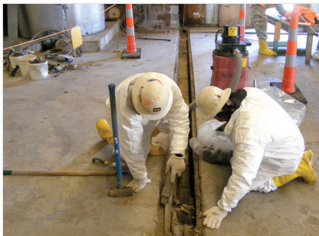
Futura Building 4 Raceway Decon
