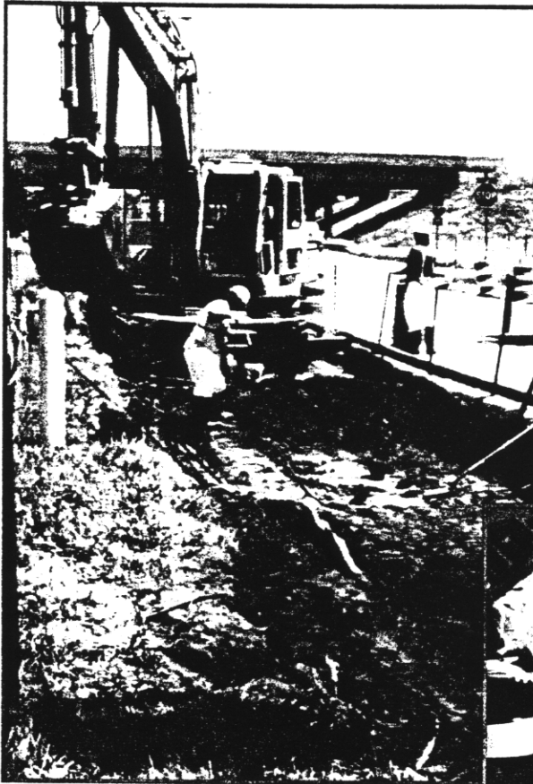
Above: Workers excavate contaminated soil near the intersection of Frost and Hazelwood avenues. I-170 crosses in the background.
