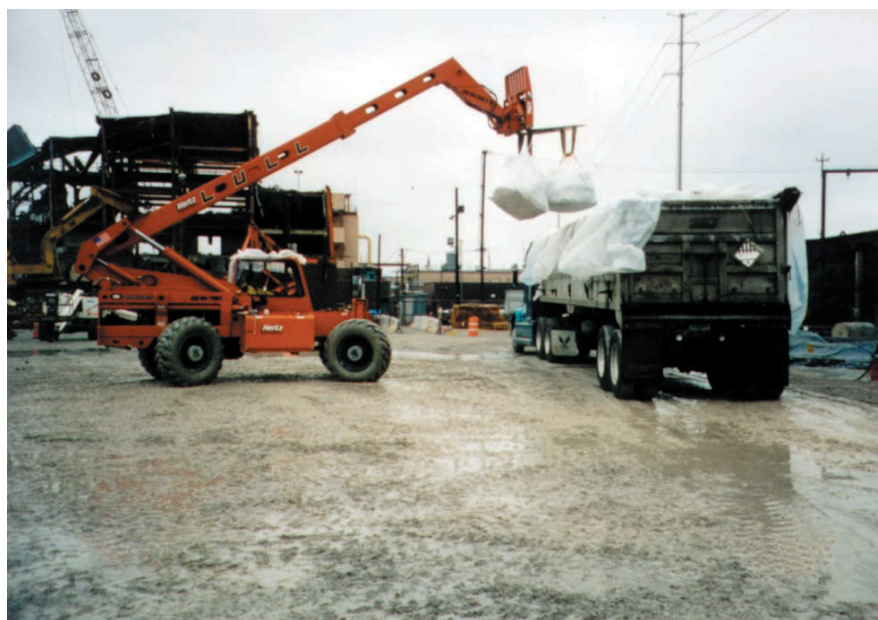
Loading material removed during preparation of buildings for demolition
