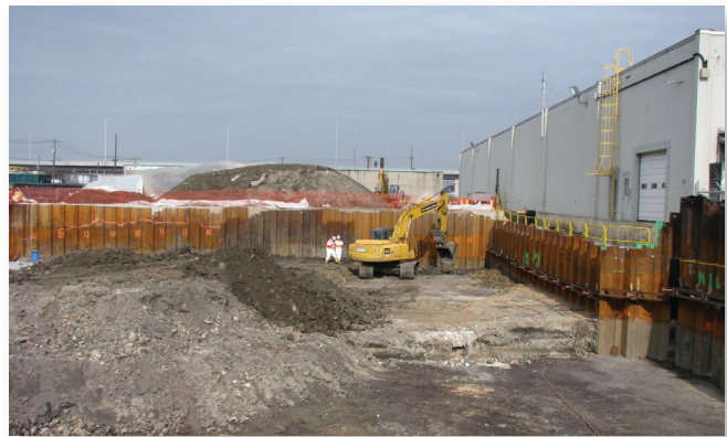
The final phase of cleanup on Mallinckrodt's Plant 6 West Half is well underway. Sheet piling forms walls around the excavation.
