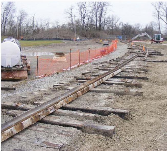
Removal of HISS Railspur
