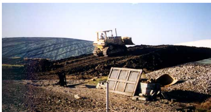
Construction crews grade soil for rail spur at the HISS site. Excess soil is temporarily stockpiled between the main and supplementary storage piles.
