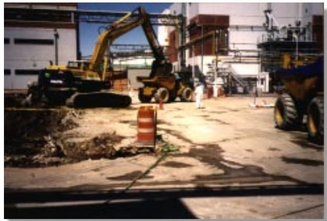
Excavators load material from the Plant 2 remediation work into trucks which transport the covered material to the SLDS railspur.
