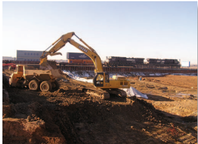
To position the site for completion in 2007, SLAPS contaminated soils will be stockpiled onsite beside the railcar loading area.
