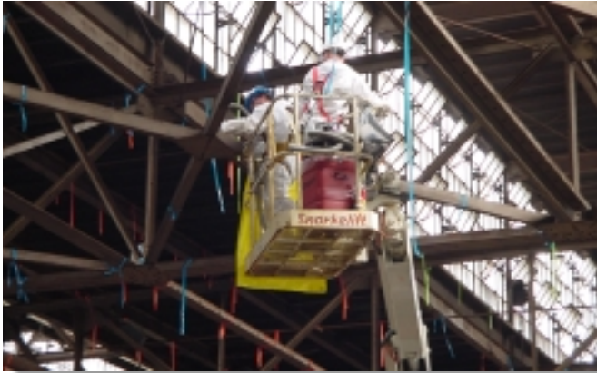
Uranium-contaminated dust at the Madison Site was vacuumed and scraped from overhead structures.
