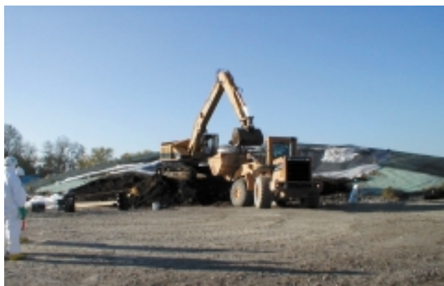
Twenty years after its initial creation, the removal of the Main Pile from HISS has begun. The pile contains approximately 25,000 cubic yards of soil.
