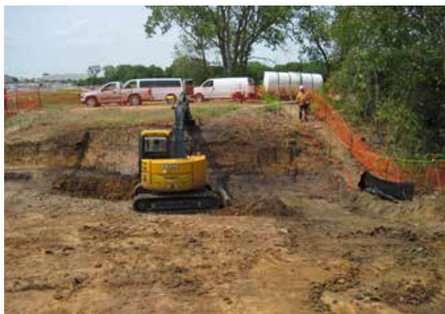
Ballfields Phase 2 Excavation
