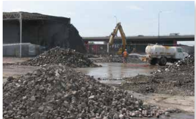
Building 101 Demolition – St. Louis Downtown Site
