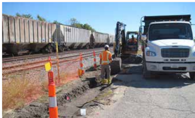
VPI6 Eva Loadout Remediation
