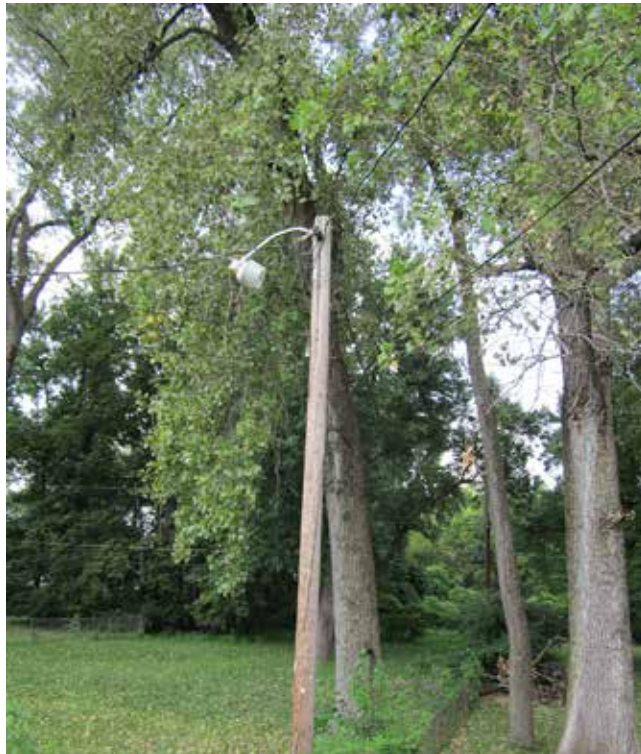
Extensive preparatory work must be done before USACE begins remediation at the Palm Drive properties.
