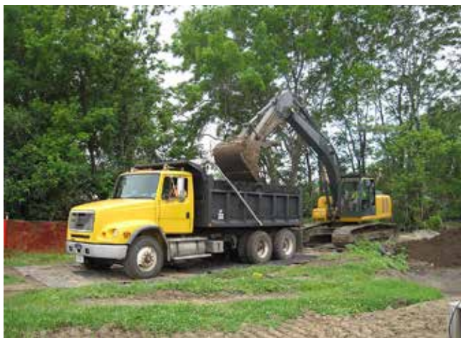
Remedial Activities at Duchesne Park in the city of Florissant.
