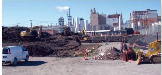
Building 101 looking west from the northeast corner - SLDS
