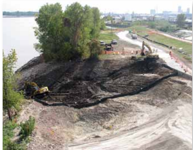
Remediation and restoration at city property east of the levee
