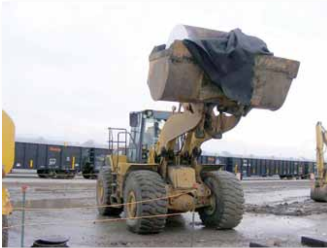
Contaminated material removed from SLAPS
