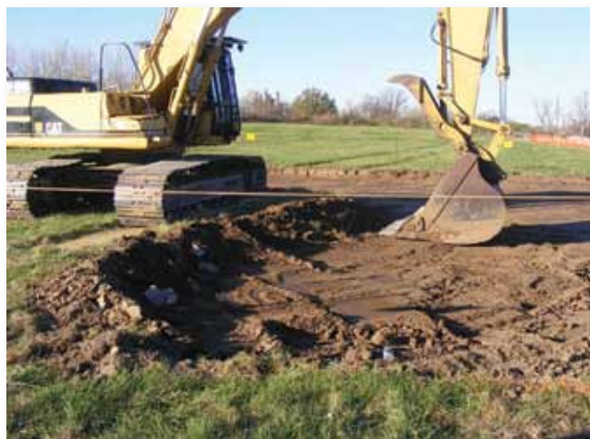
Removal of contaminated soil at the Ballfields area
