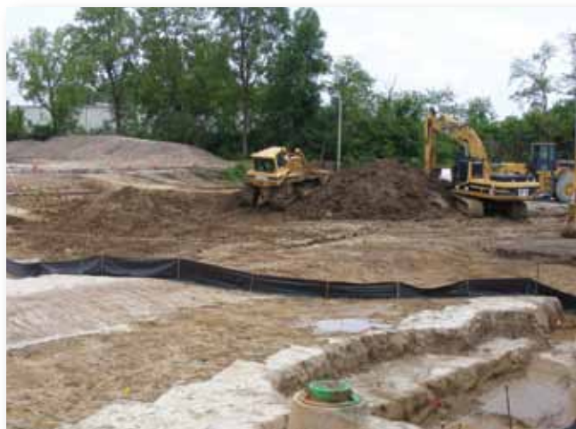
USACE completed remedial activities at VP-02L in FY10.
