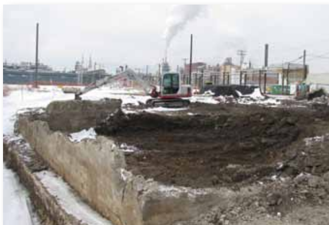
Excavation of the Plant 7 Hazardous Waste Storage Area continued during FY10.
