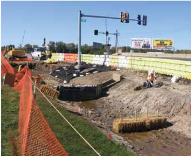
Remediation proceeds along the McDonnell Boulevard Right-of-Way.
