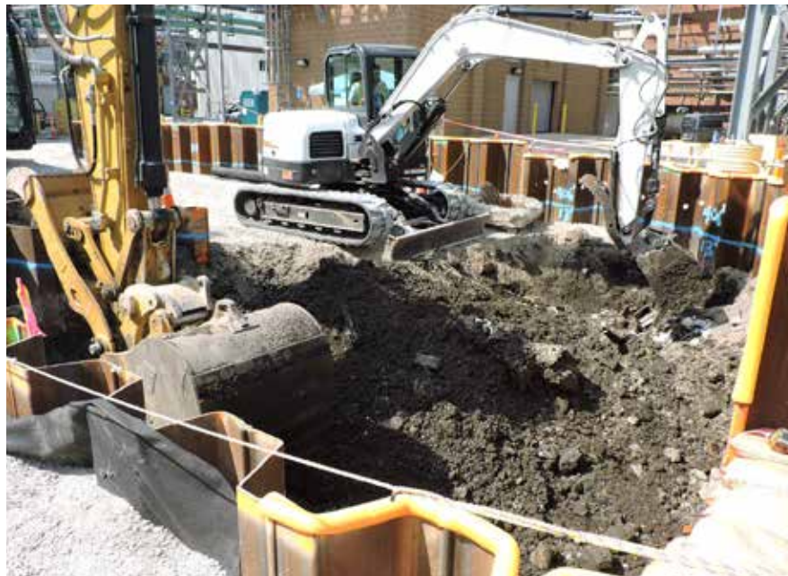
The FUSRAP team excavated contaminated soil at former Building 17 at SLDS.
