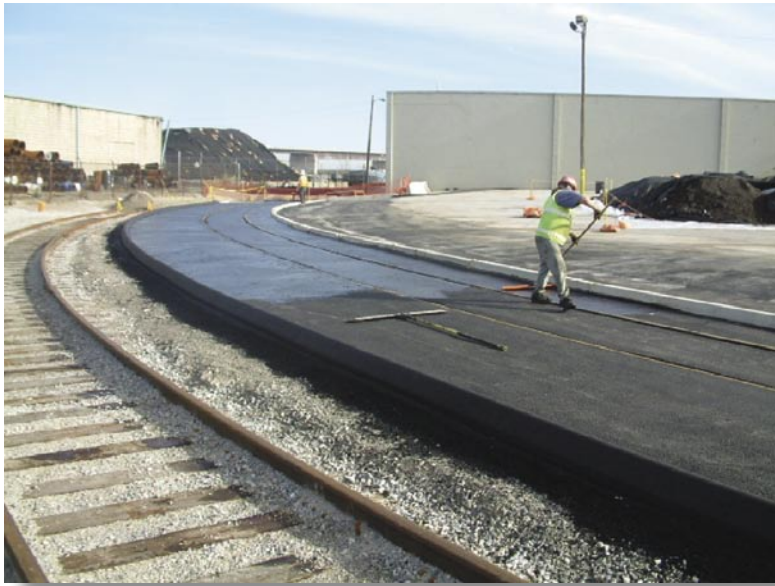
Applying sealant to the Plant 6 rail spur.
