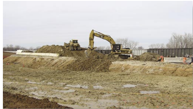
Final yards of contaminated soil at SLAPS are excavated.
