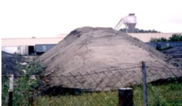
The spoil piles were recently sprayed with a gray polymer-type coating, which has stabilized them until their scheduled removal this fall.
