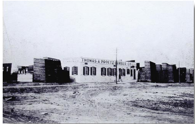
The Thomas & Proetz office building was constructed in 1903. This photo from Angelrodt Street was taken in 1910.
