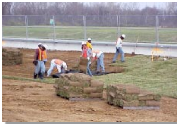
Crews lay sod as part of the site backfill and restoration process upon completing the cleanup of the East End Extension.
