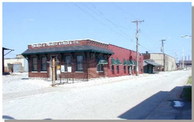
DT-10 remediation activities began in November 2004.
