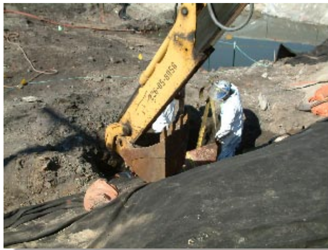
Repair of a sewer line in Plant 6WH Phase I.
