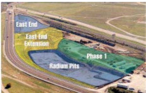
The long, thin finger of the East End Extension in the drainage ditch along McDonnell Boulevard will be removed next summer to avoid potential water management problems during wet winter months.
