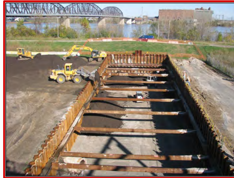
Extensive use of sheet pile
