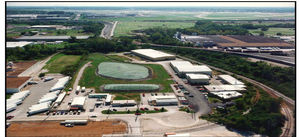
2000 Photo of the HISS storage piles and Futura buildings on Latty Avenue
