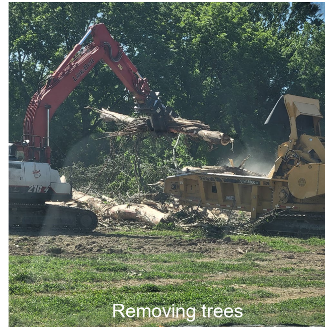
Clearing trees and building road
