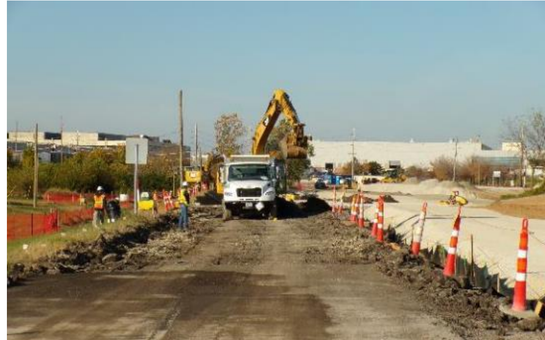
Remedial activities on McDonnell Boulevard
