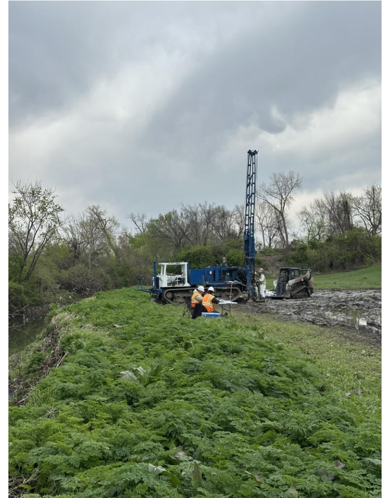
Drilling groundwater wells along Coldwater Creek
