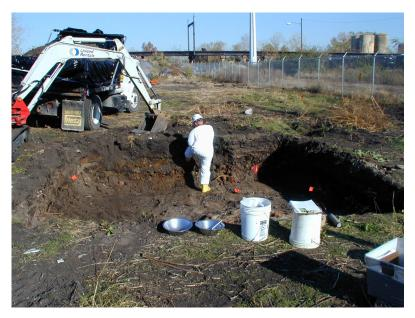
are marked and excavated. This is referred to as "guided excavation" since limited portions of the work area require excavation to a deeper elevation to achieve the selected remedy. Precision excavation minimizes the potential for cross-contamination of clean areas.
