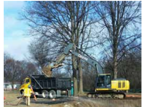
Remedial activities at Duchesne Park are now complete.
