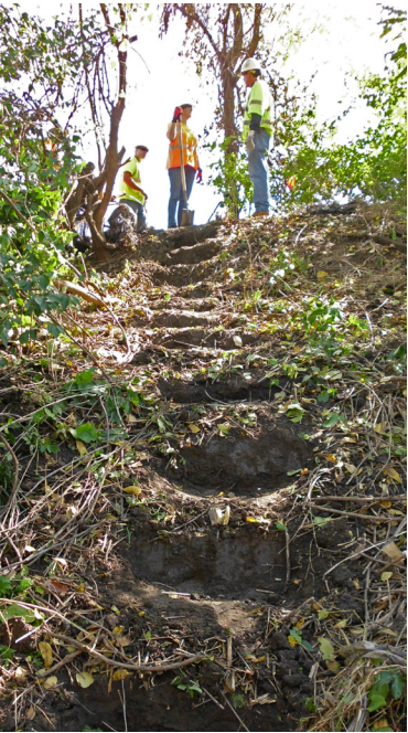
Project scope, scheduling, bad weather, or difficult access can lengthen the CWC sampling timeline. Additional actions may also be required. For example, a crew may need additional time to clear away heavy brush or cut steps into a steep embankment.
