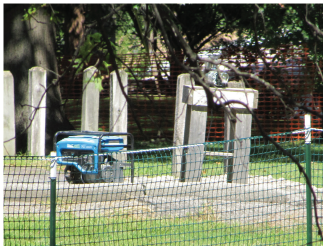
Inside an access-restricted FUSRAP work site, a generator on the left powers an air sampling unit on the right.
