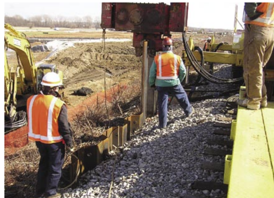
Crews are installing sheet piling along the Norfolk Southern Corporation rail line from a rail-mounted crane. Sheet piling is being installed to maintain the stability of the rail line during upcoming cleanup activities.
