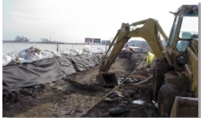
Since October 1997, the USACE has removed 112,600 cubic yards of contaminated material from SLAPS.
