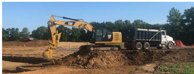
The contractor removes low-level radioactive material from Area 1 of the former Ballfields Phase 2B in North St. Louis County with a track-mounted excavator Wednesday, July 18, 2018.
