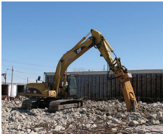
Demolition of SLDS 700 Pad
