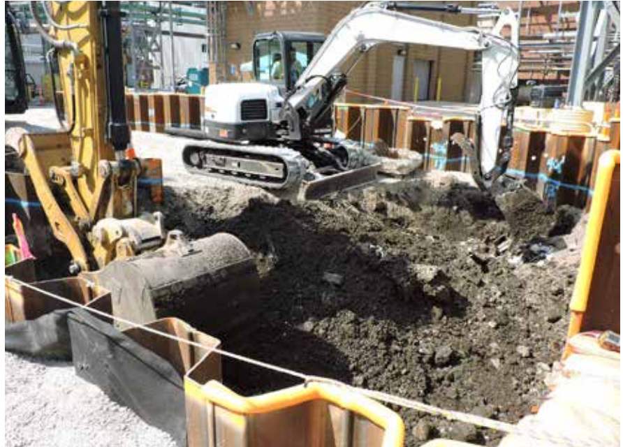
The FUSRAP team excavated contaminated soil at former Building 17 at SLDS.
