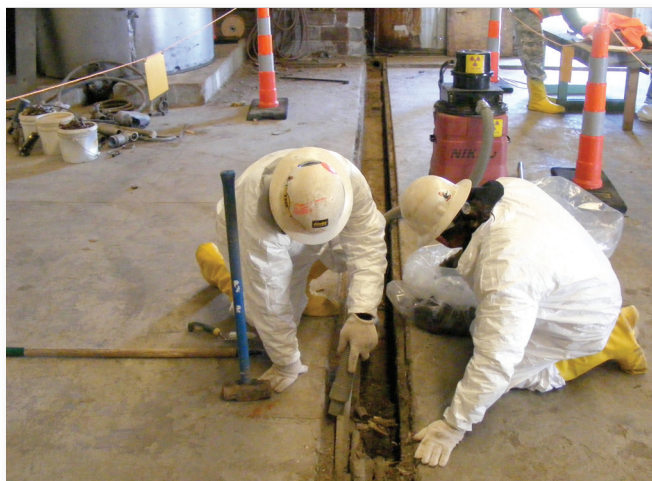
Futura Building 4 Raceway Decon
