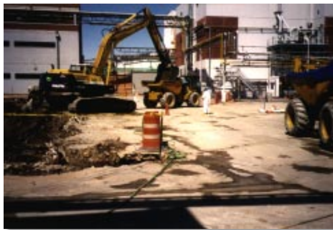
Excavators load material from the Plant 2 remediation work into trucks which transport the covered material to the SLDS railspur.
