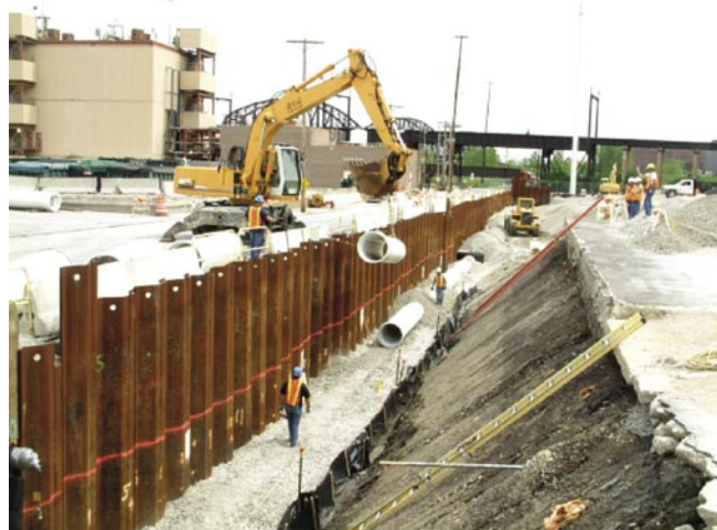
Sheet pile retaining wall preserves Destrehan Street stability during Plant 7N/7S remediation.
