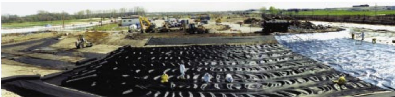
To prevent sediment transport, the basin is lined with a geomembrane fabric and crushed stone. Workers are shown installing the fabric. The fabric creates a barrier between the contaminated sediments, which settle out of the storm water run-off, and the soils below the basin.
