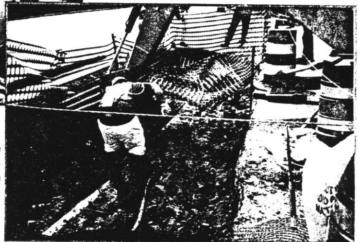
Above: Workers view a fresh cut made by an excavator. Right Only old-fashioned hand excavation will do near a utility conduit.
