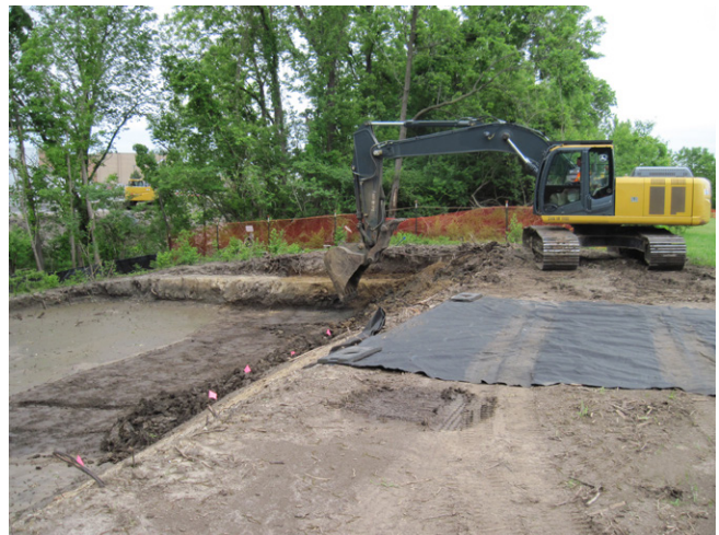
To date, USACE removed over 1,500 cubic yard of contaminated material from Duchesne Park.
