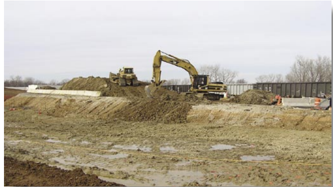
Final yards of contaminated soil at SLAPS are excavated.
