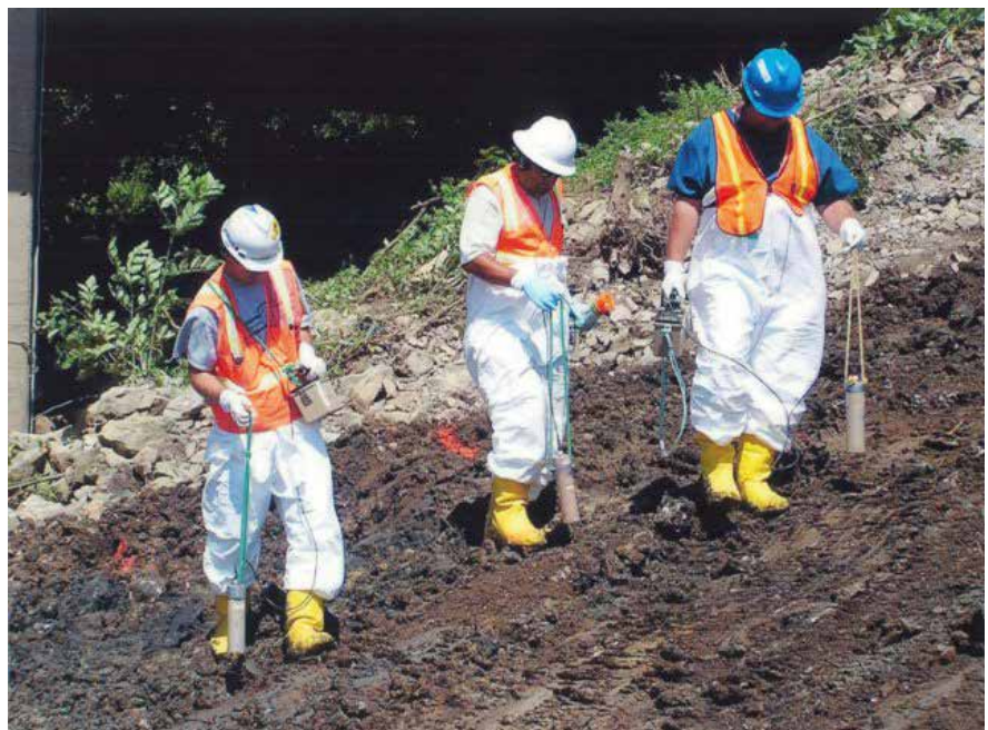
USACE protects public health and the environment by removing low-level radioactive contamination generated by uranium processing from the 1940s and 1950s. Workers use survey equipment to confirm cleanup.
