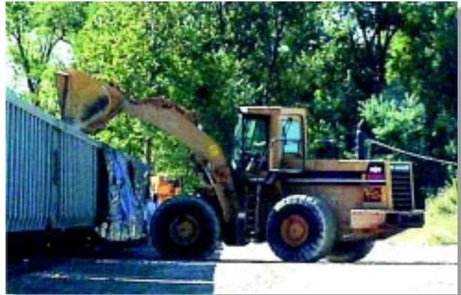
Removal of the final stockpile at HISS is nearly complete. Of the estimated 25,000 cubic yards comprising the Main Pile, roughly 20,200 cubic yards have been removed.
