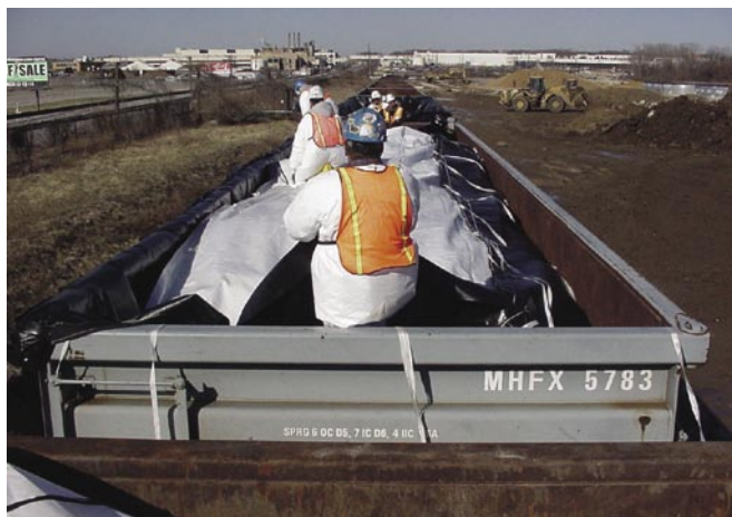
USACE follows U.S. Department of Transportation regulations to package and transport contaminated materials from the FUSRAP sites.
