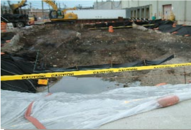
At the St. Louis Downtown Site (SLDS) crews had to deal with old concrete foundations, overhead and underground utilities and water infiltration during remediation of Plant 6W Half Phase I.
