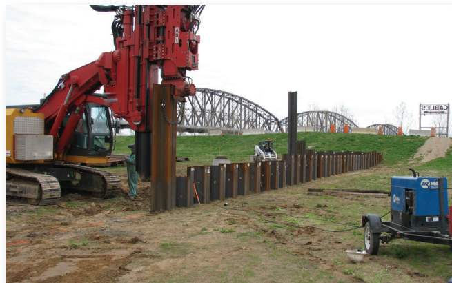
Heavy pile-driving equipment is used to initiate the sheet pile protection for the City Property Vicinity Property at SLDS.
