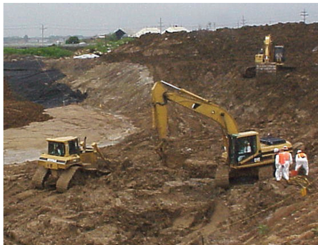
More than 80,000 cubic feet of soil was excavated to complete Phase 1.
