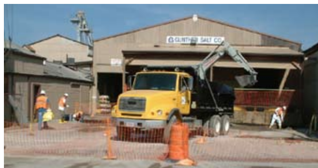
Excavation activities at Gunther Salt North and South resulted in the removal of 2,826 cy of contaminated material to an out-of-state licensed/permitted disposal facility.
