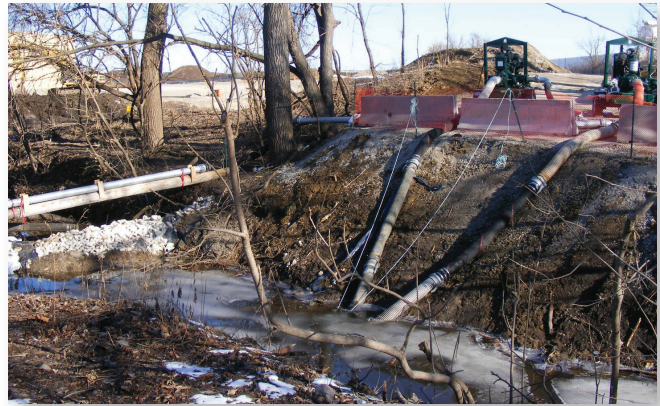
Two large pumps divert Coldwater Creek flow around an excavation at the Norfolk Southern Vicinity Property in North County.
