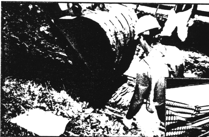
Above: Workers view a fresh cut made by an excavator. Right Only old-fashioned hand excavation will do near a utility conduit.
