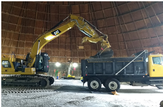
An excavator operator dumps a bucket of contaminated soil into a dump truck at Gunther Salt Dome recently.
