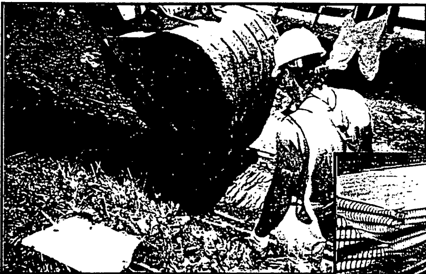
Above: Workers view a fresh cut made by an excavator. Right Only old-fashioned hand excavation will do near a utility conduit.
