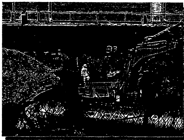
Excavation of Plant 2 concluded in April with the removal of approximately 10,200 cubic yards of material.
