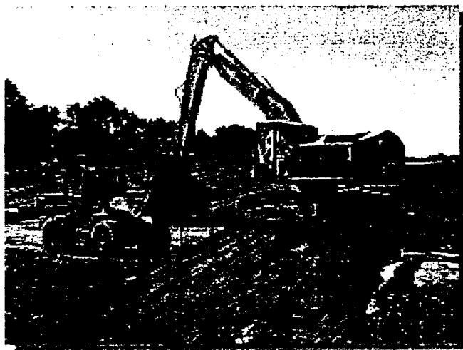
The excavator (shown above) is moving material from the HISS Supplemental Pile into a front end loader, which takes the material directly to the railcars.
