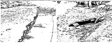
April 17, 2002. A break in a water main washed away soil and gravel from under a road causing it to sink. USACoE personnel provided HP support to construction crews in preventing further spread of contamination that could result from the repairs.
