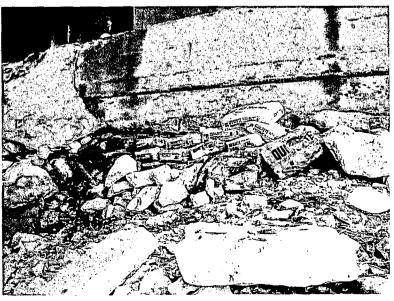
Coldwater Creek has been flooded several times the past two months. The top photo was taken from the railroad bridge crossing the creek and bordering SLAPS. A cavity under the foundation of the bridge, approximately 18 feet wide, 2 feet high, and 1.5 feet deep, resulted as soil and rock were swept away by the creek. Norfolk Southern is attempting to prevent further loss of soil however further repairs with assistance from the USACoE may soon be needed.
