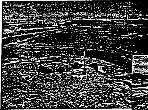
Right: Deep pockets appear in the excavation. Currently, these pockets are dry but in a heavy rainfall, they will hold contaminated water until it can be treated and released.
