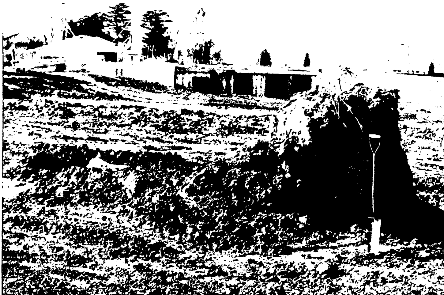
Figure 6.—Construction on Urban land-Harvester complex, 2 to 9 percent slopes. Mound in right foreground indicates the amount of cutting at this site.
