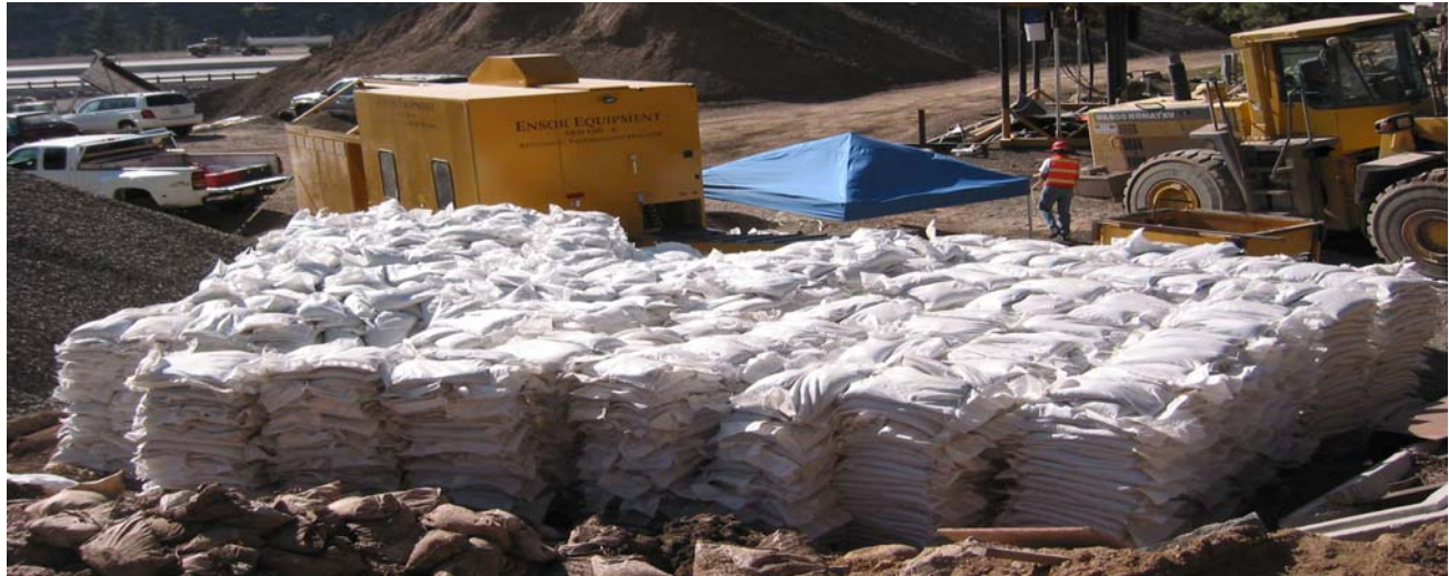
Granite Construction I-80 Project, Truckee, CA
