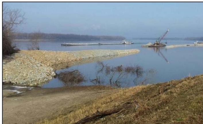
Restoration of the Bankline, Len Small
