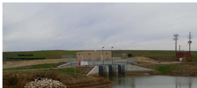
New Chain of Rocks Pump Station
